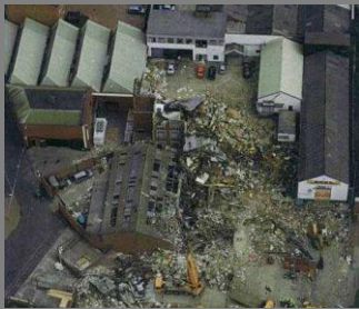
Nine died and 45 people were seriously injured in the 2004 explosion Photo HSE
