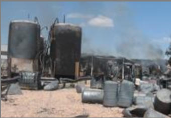
The scale of the fire damage
