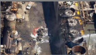
Sky7 HD flew over the Chevron refinery in Richmond to take a look at the fire damage.
