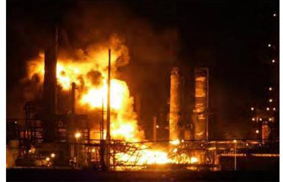
CSB determined that the propane fire resulted from water freezing and cracking an idle section of process piping.
