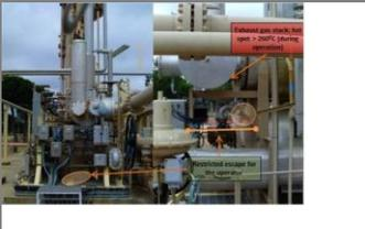
Front and side view of the dehydration unit. TEG inlet design aiming to hot spot.
