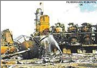
**Fig 10 - On 1 June 1974, a vapor cloud explosion destroyed the Nypro cyclohexane oxidation plant at Flixborough.**
