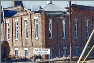
An explosion blew off a corner of the one-story brick building's roof and wall, sending bricks and debris onto Burlington Northern railroad tracks.
