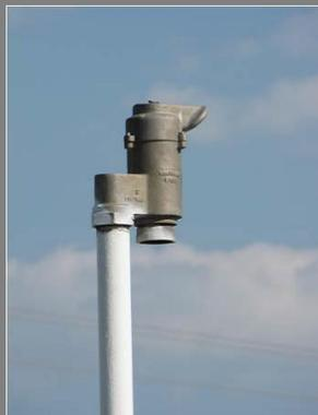
The pressure Vac Vent should be inspected monthly and maintained during freezing conditions
