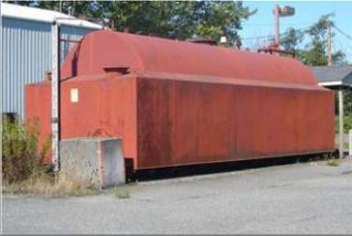
Aboveground flammable and combustible liquid tanks are produced in a variety of shapes. Tanks are permitted to be of any shape, size or type consistent with sound engineering practices. They do not have to be listed by an independent testing agency. (See Coffee Break Training FP-2010-21 for a description of “listed” products.) The most common shapes of steel tanks are cylindrical horizontal, cylindrical vertical and rectangular.
