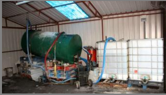
The illegal diesel plant found in Newry. (© HMRC)
