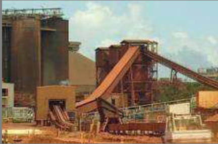
About 70,000 litres of unleaded petrol leaked from an old tank at the Alcan plant.
