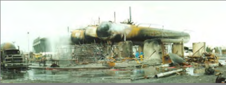
View of the LPG terminal after the explosion. Note: damaged manifold and pipes (centre left), Tank No 1 missing (centre right), remains of the destroyed LPG Road Tanker (far right) and discharge pipes from the PRVs on the top of each tank
