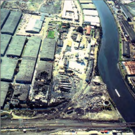
Aerial view of the BORAL Gas site after the fire.
