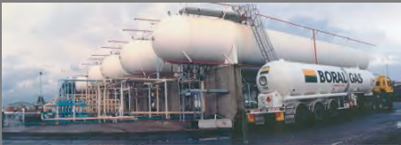
View of the LPG terminal before the explosion. Note: Red drencher pipes above and below each tank, and the LPG Road tanker in a similar position to that of the night of the explosion
