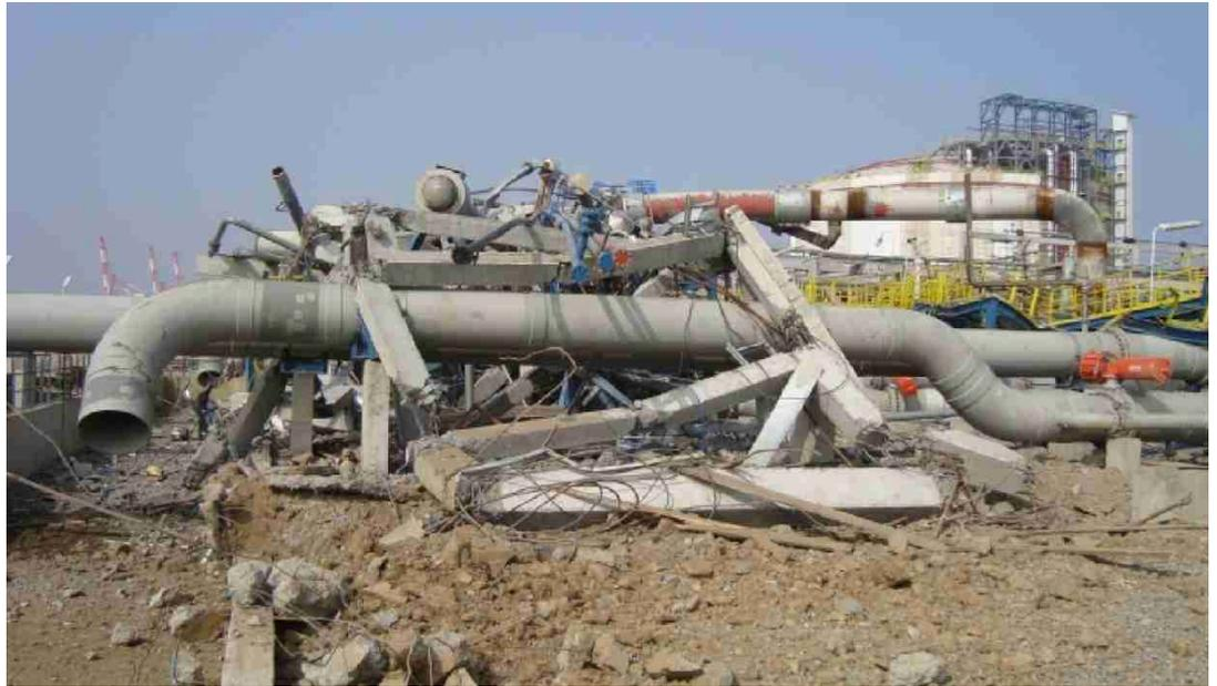
The explosion occurred during a pressure test of the equipment, according to the city government media office. Workers were pumping air into a gasifier when, some 500 meters of the piping network burst into fragments, buckling cement crossbeams. The cause of the rupture was still under investigation, the Shanghai Commission of Safety Production said.
